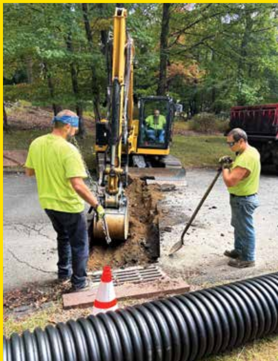
Highway Department employees working on a drainage project in town.
